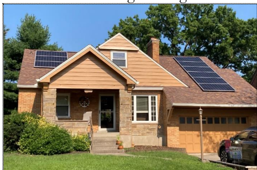
A 2021 Silverton Solar Now home is now net neutral
